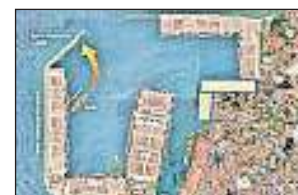
WCT is strategically located next to a $500-million Chinese-run container jetty
